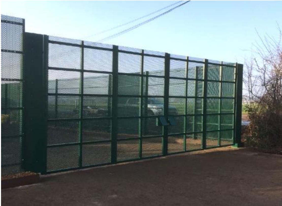
Example of SEAP Class 2 fence from catalogue
