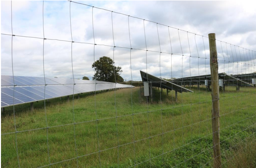
Example of weldmesh security fencing at solar farm
