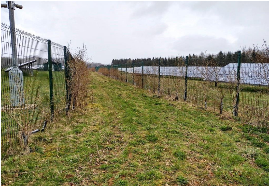
Example of weldmesh security fencing at solar farm
